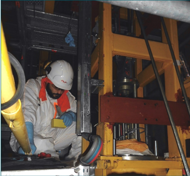
Figure 18. Carrying out work on the containment manipulator.
