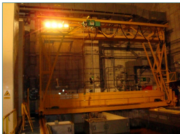
Figure 1. Overview of the spent fuel pool bridge.
