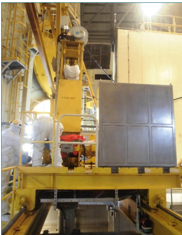
Figure 9. Renovation work on the containment manipulator crane.
