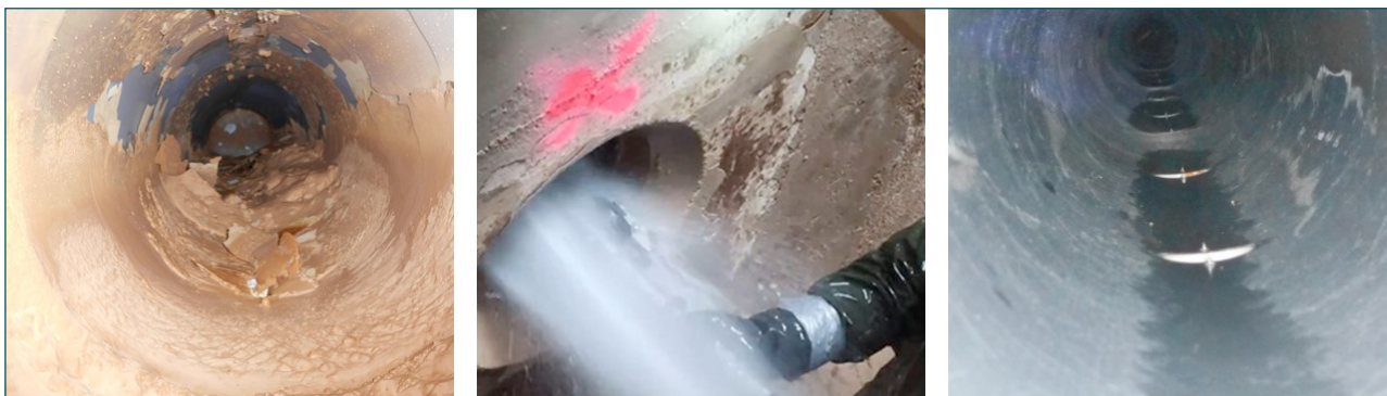
Figure 7. Initial state of pipes, cleaning process and final state.
