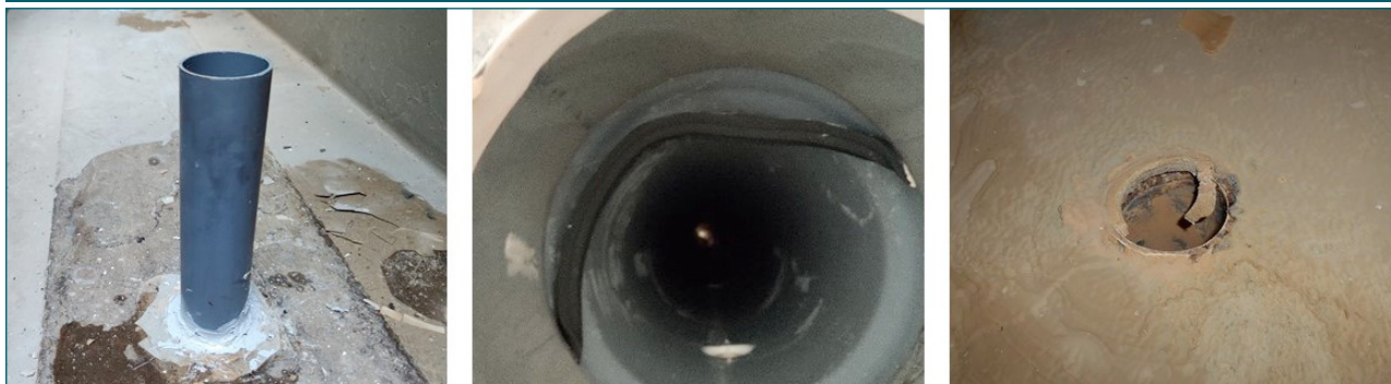
Figure 9. Images of other maintenance activities.
