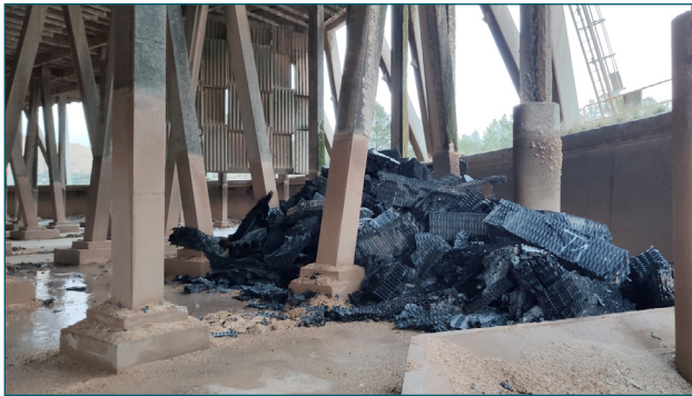
Figure 10. Removal of the fill packs.
