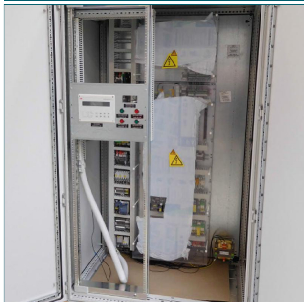
Figure 5. MAEX®, synchronization and operator panel in transportation cabinet.
