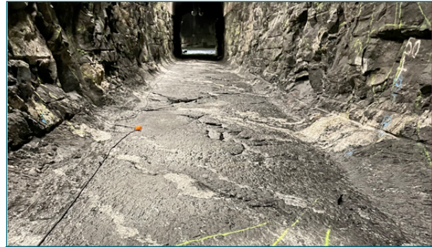
Figure 7. A deposition tunnel in the spent fuel repository, picture Timo Saanio.
