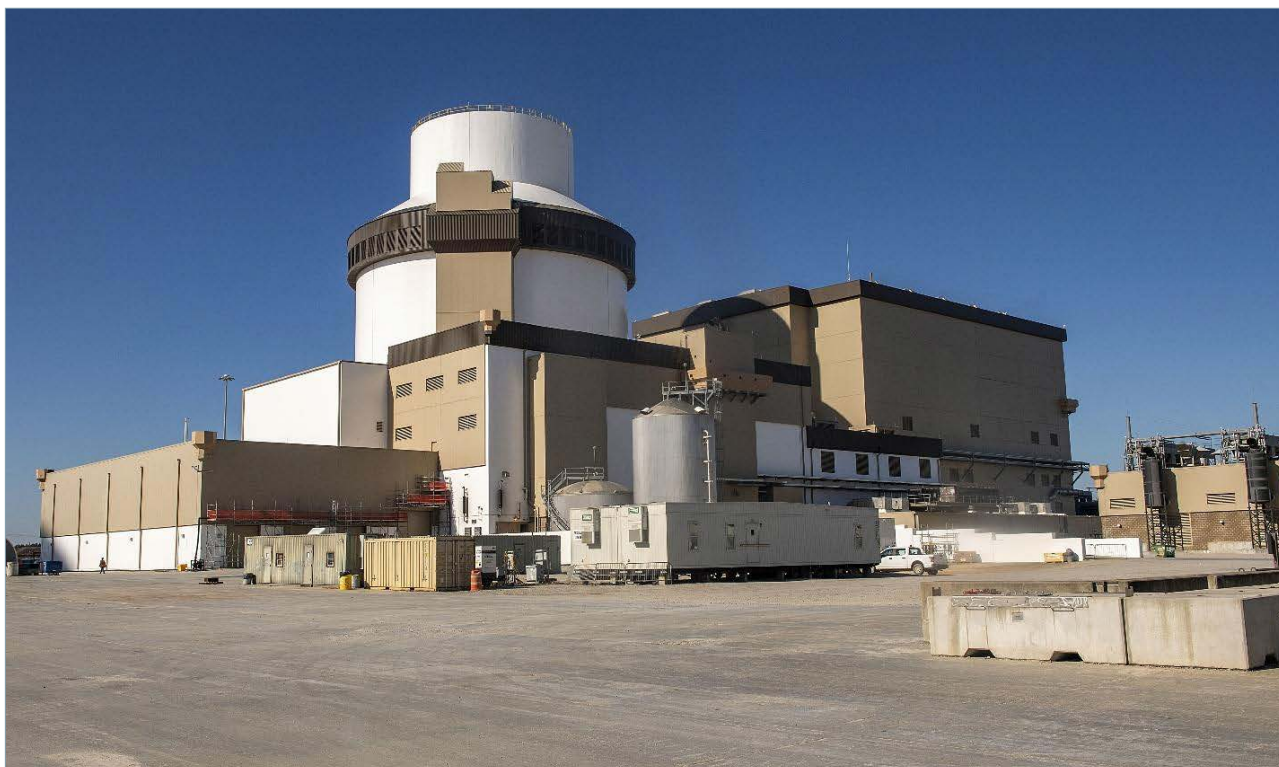
Figura 5. Reactor Nuclear WestinghouseVogtle 4 AP1000 en Georgia.
