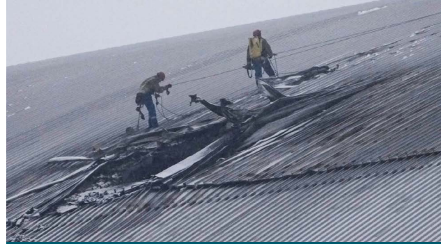
Figure 3. Drone strike on the New Safety Containment of unit 4 of Chernobyl NPP.
