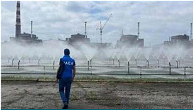
Figure 2. Open sprinklers as link for the crucial cooling chain at Zaporizhzhia NPP.
