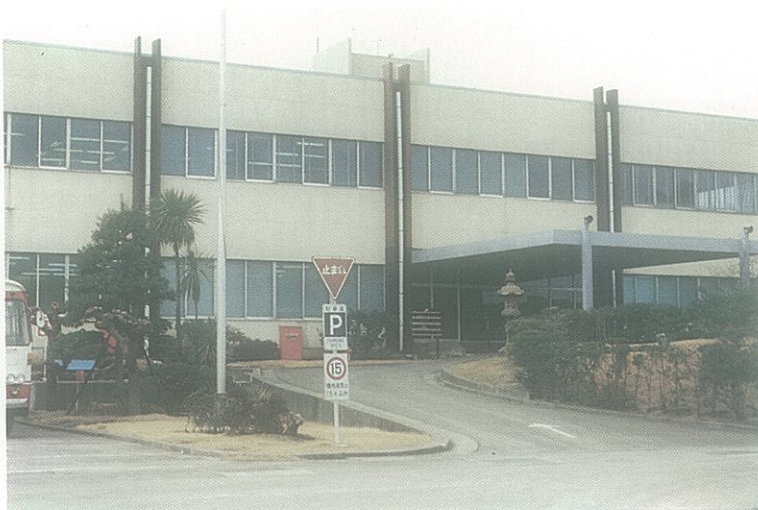
Located in Kurihama, Japan, JNF is jointly owned by General Electric, Hitachi, and Toshiba.
