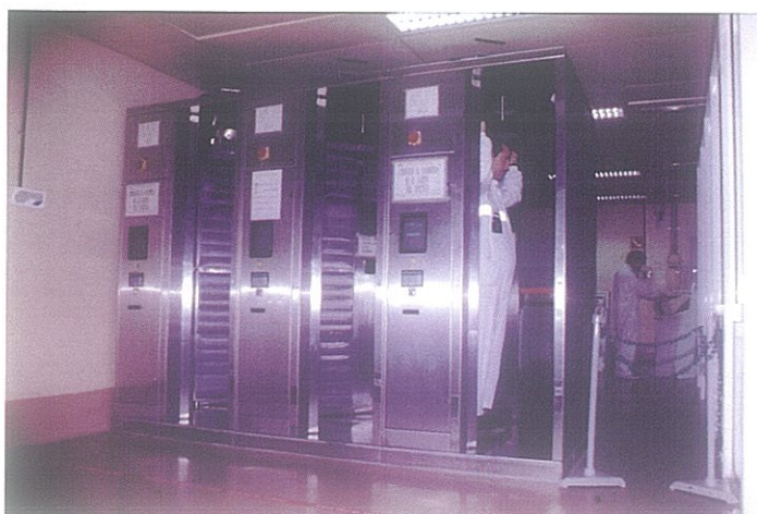
A radiation Protection control and check point
