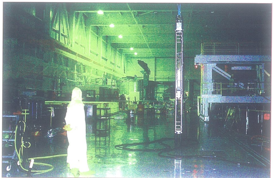
Teide-2 ready for inspection on refueling platform.
