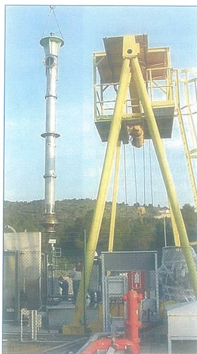
Installation maneuver of one of the new Essential Service Water pumps.
