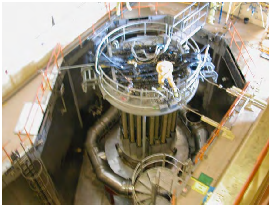
Activities in refueling cavity.
