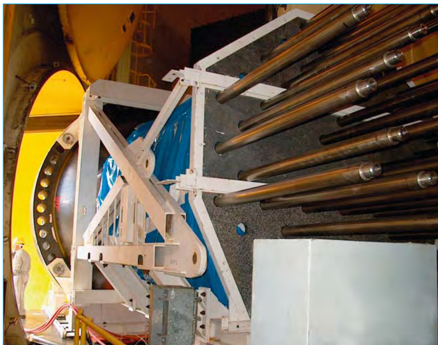
Reactor vessel head replacement maneuver.
