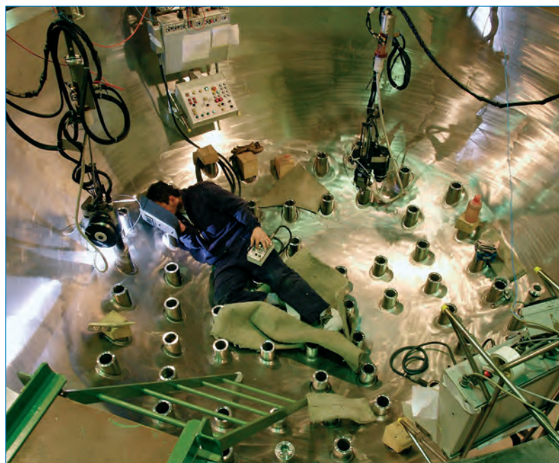
Hoy. Soldadura Automática CRD a Tapa. / Today. Automatic Welding CRD to Head Cap.
