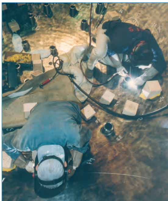
Antes. Soldadura Manual CRD a Tapa. / Before. Manual Welding CRD to Head Cap.
