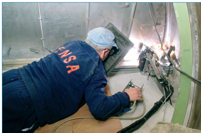
Hoy. Soldadura Automática Placa Divisoria. / Today. Automatic Welding of Partition Plate
