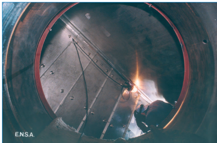
Antes. Soldadura Manual Placa Divisoria. / Before. Manual Welding of Partition Plate
