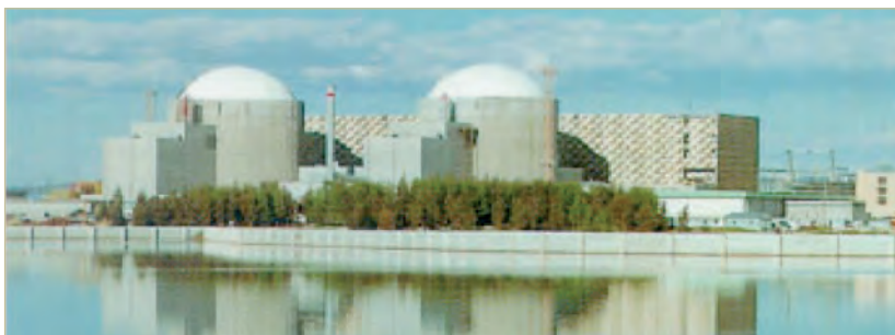
Central Nuclear de Almaraz (PWR, Westinghouse, 2X980 MWe).
