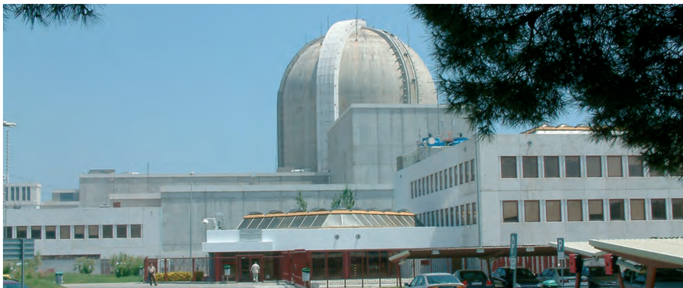
Central nuclear Vandellós II / Vandellós II Nuclear Power Plant
