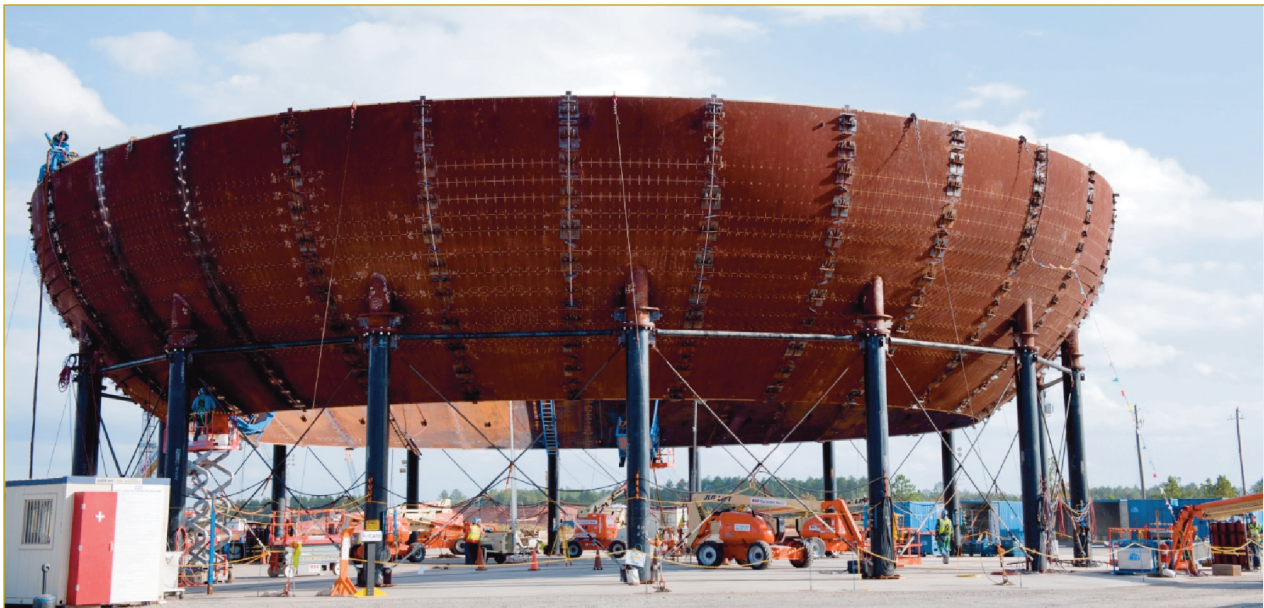
Upper section of Vogtle Unit 3 containment vessel lower head fastened to assembly and welding stand. November 3, 2011 ©2011 Southern Company, Inc. All rights reserved.
