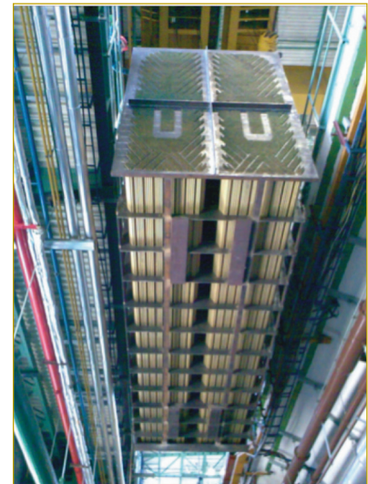
Detail of Open Top Installation of TG31 condenser bundles. Notice accurate constructability design.
