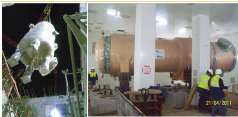
Picture 7. Installation of several Flamanville Safety Class HX (Open Top and Non Open Top).
