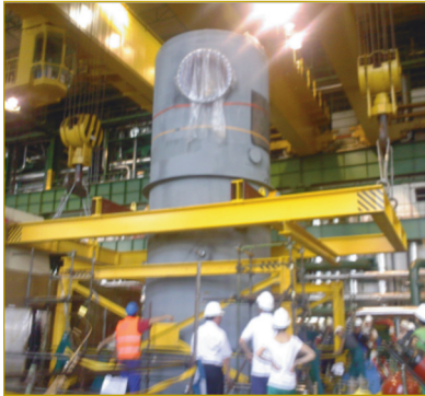
Rigging for new MSR Bohunice.
