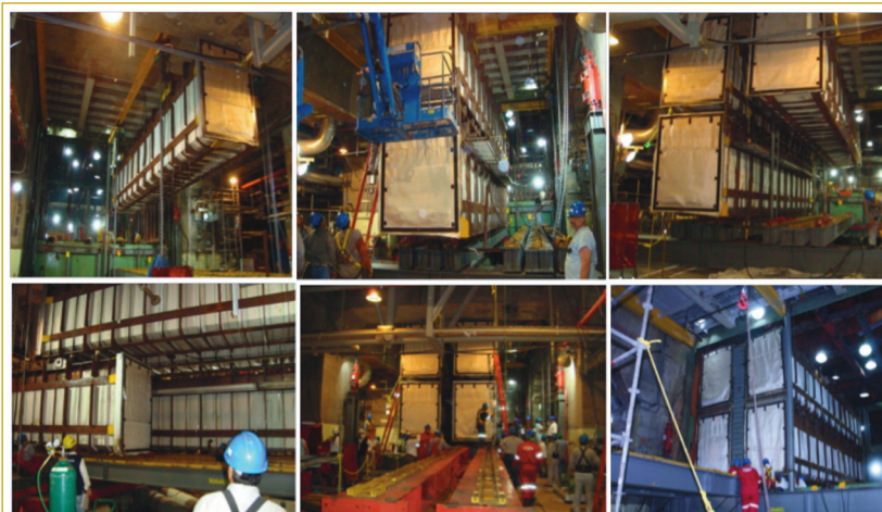
Laguna Verde Unit 2 Condenser Installation sequence using Modularization scheme of construction (from top left to the right upto lowest right picture).
