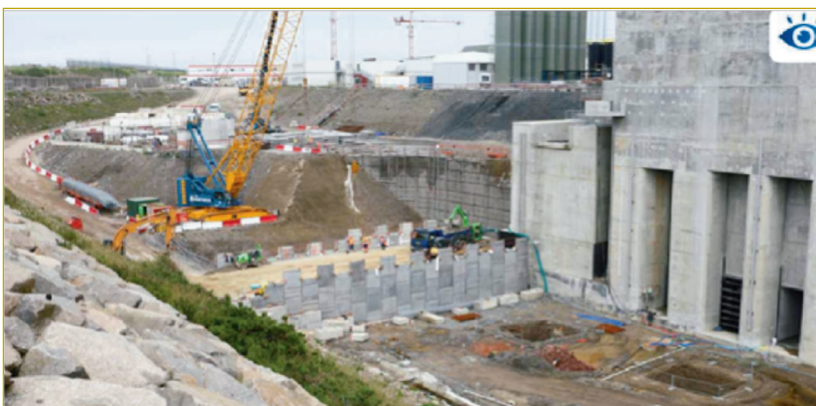
Picture 8. Circulation Water Channel Construction. Flamanville 3.
