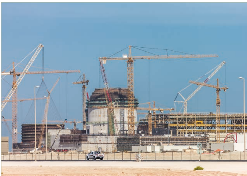
Figure 1. Construction of Unit 1 of the Barakah Nuclear Power Plant in the UAE. (Photo: ENEC, UAE).
