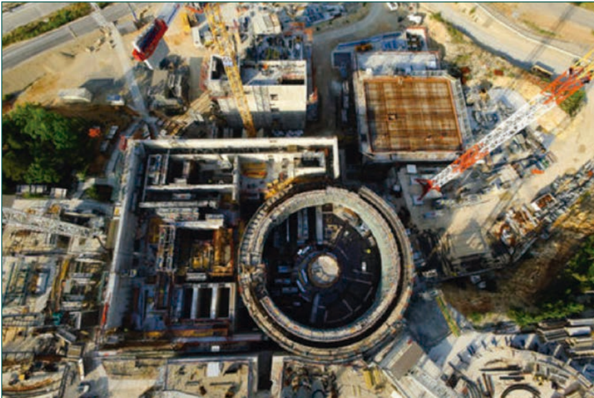
Construction of the Jules Horowitz Research Reactor in Cadarache (France).
