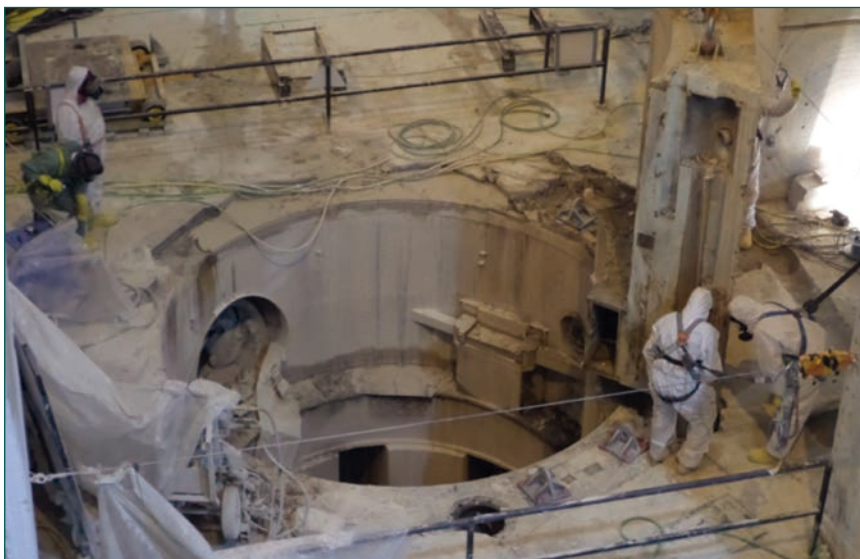
Source: Enresa. José Cabrera NPP dismantling, cutting of concrete.
