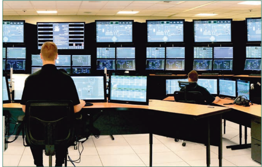
Figure 6. Photograph of NuScale multi-module control room simulator.
