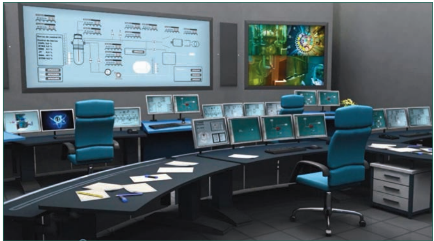
Figure 4. Control room with a distributed software system.
