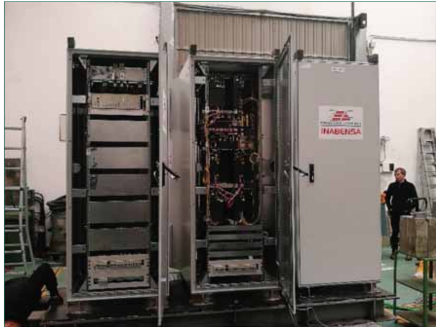
Figure 3. EUT cubicles mounted on the shaking table at the seismic qualification test.
